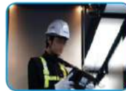
■ Adjusting the camera angle at the elevator
